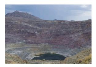
Mines frequently dig pits that pierce the groundwater table, creating a pit lake after mining ends and dewatering pumps are shut down. As the pit lake evaporates in the Sonoran Desert heat, groundwater from the surrounding area is drawn into the pit. Pulling water into the pit reduces the likelihood of dangerous contaminants from spreading outward into the aguifer.
